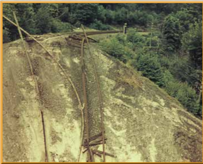
Devastation at the Devils Hole railroad crossing led to catastrophic damage downstream. Here the railroad tracks are seen hanging in air.
